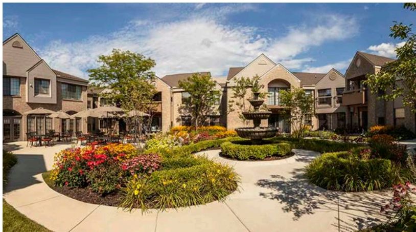
An example of courtyard style Senior Living Facilities
