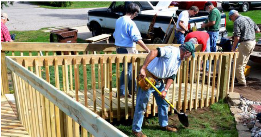
VOLUNTEERS BUILDING ACCESS RAMP
